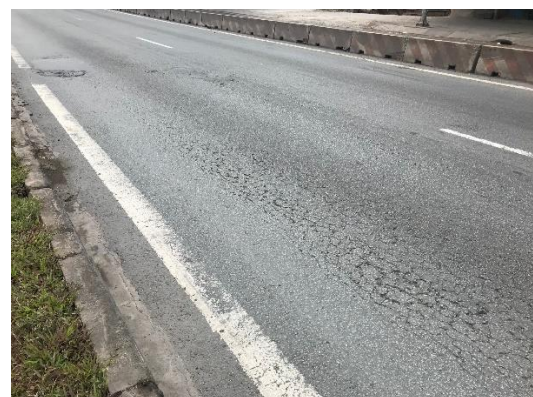
Fig. 1. Fatigue cracks and pothole in National Highway 1A, located near Thu Duc District, Ho Chi Minh City, Vietnam [9].
