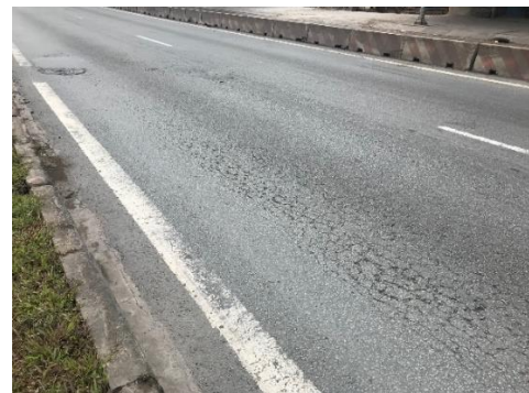
Fig. 1. Fatigue cracks and potholes in National Highway 1A, located near Thu Duc District, Ho Chi Minh City, Vietnam
