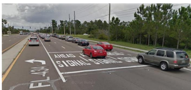
Figure 3. Pavement marking countermeasure
